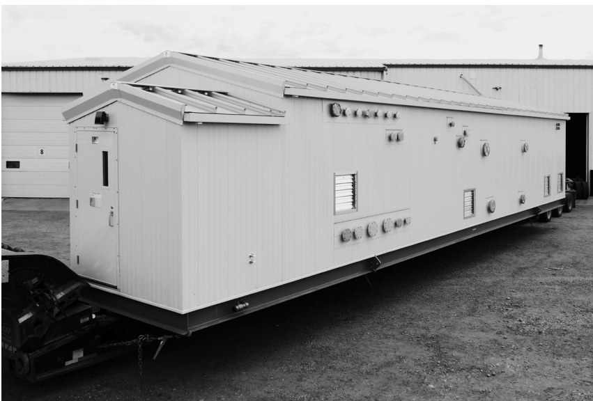
The building package leaving Ultimate Fabrication. The 15 m (150 ft) long trailer weighed 50 tons (110,000 lbs).
